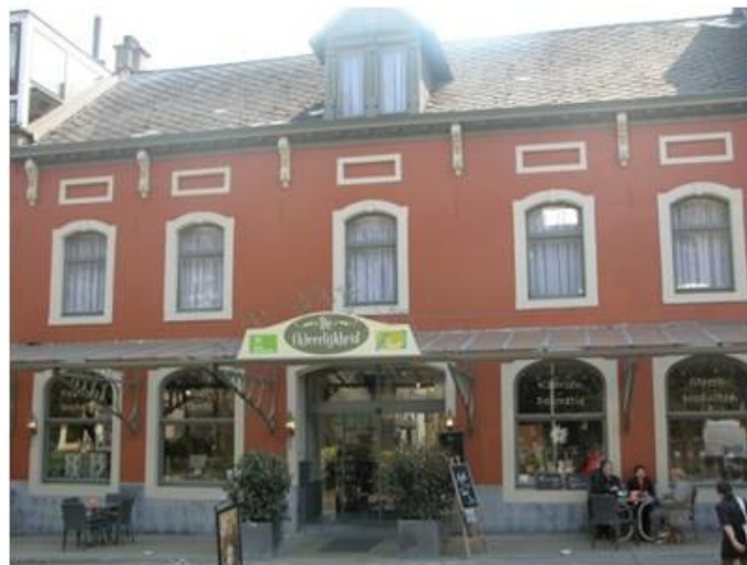
Photograph: Building after renovation.
