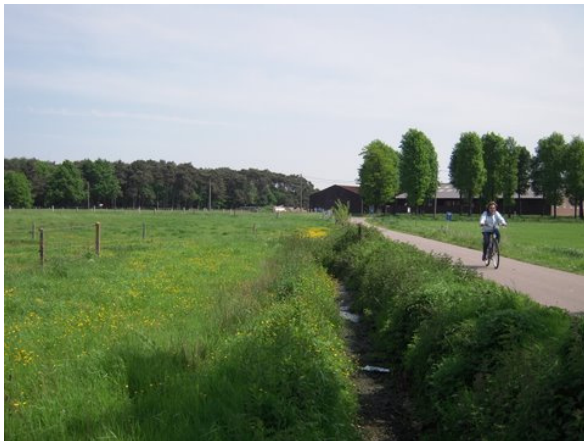
Photograph: Embankment along the cycling path.
